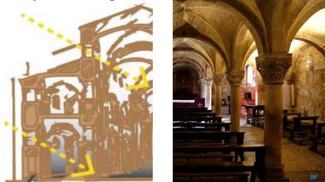
Figure I.6 St. Michele Pavia, Italy, c. 1100 - 1160 with masonry vaults required massive walls with small openings
