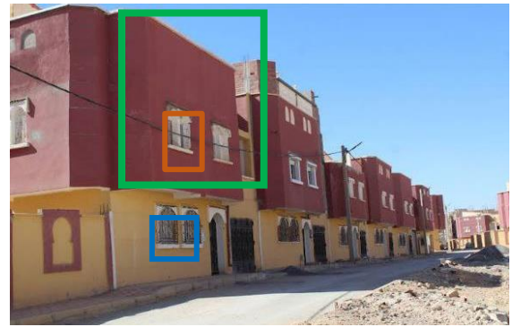
Figure 98 : Shading and sun protection elements in facade source : the writer,2025
