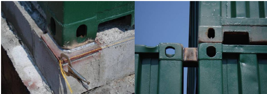
Figure 31a) Welded shipping container to base plate and (b) uncommon connection between shipping containers from Hermann (Giriunas, Sezen, & Dupaix, 2012)
