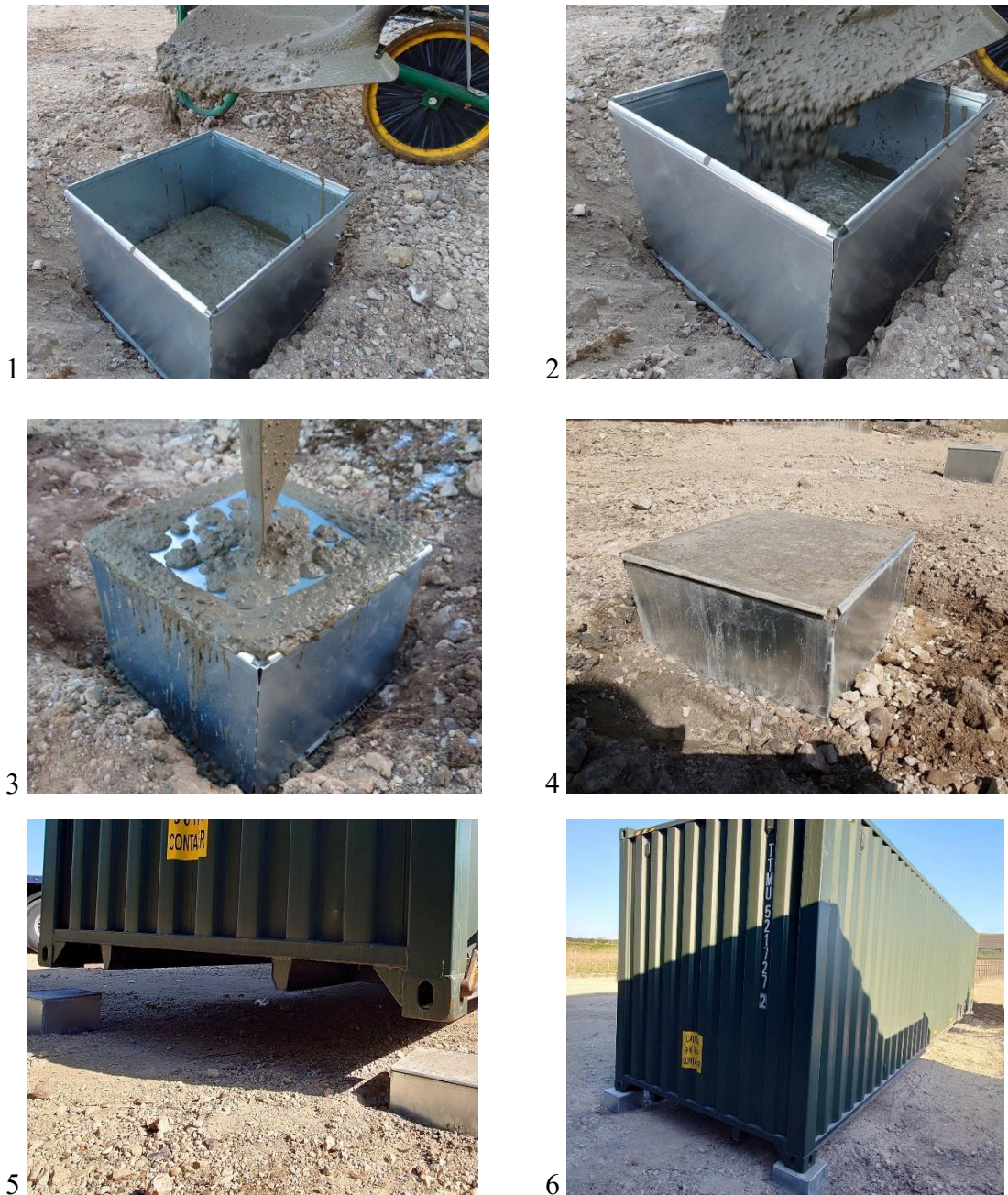
Figure 30 : Chipping Container Foundation Concrete Base Mould of 300mm sides by 220mm height ( ndooroutdoors.co.uk/products/shipping-container-foundation-concrete-base-mold )
