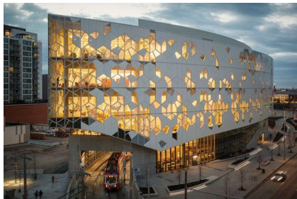
Figure 15: Calgary Central Public Library Source: www.archdaily
