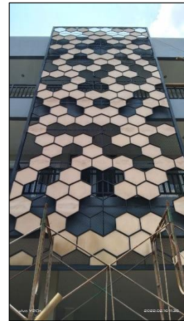
Figure 98: Façade au brise-soleil Source: Pinterest.com
