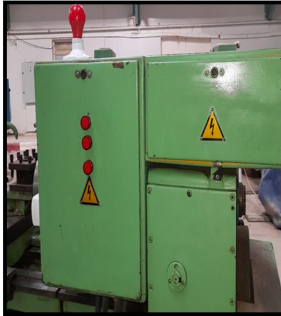
Figure III.29: Lampes témoins en cas de surcharge.
