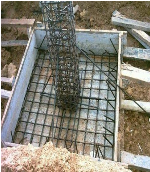
Figure 11: Isolated Footings (Point Foundations)
