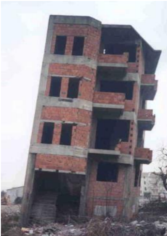
Figure 22: Tassement of Foundations
