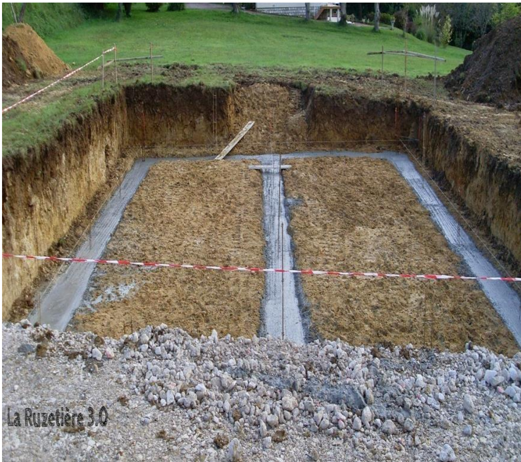
Figure 13: Strip Footings in Trenches
