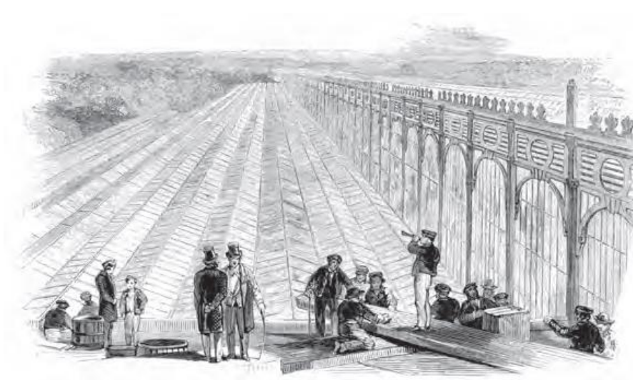
Figure IV.6. One of the technical enablers of the open space. Glass Roof of the Crystal Palace. Source: Garrido, 2023, p.75
