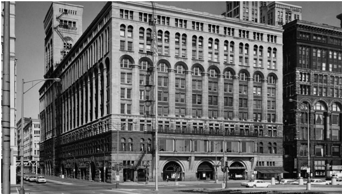
Figure VII.11. The Auditorium Building at Roosevelt College, Chicago, 1933. Source : https://www.nps.gov/places/auditorium-roosevelt-u-il.htm
