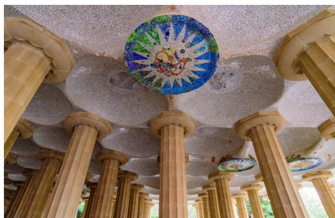
Figure VI.11. Barcelona's Park Güell: (Above-left) General view; (Above-Right) El Drac; (Below) The hypostyle hall. Source: https://www.barcelona-tickets.com/fr/park-guell/inside/
