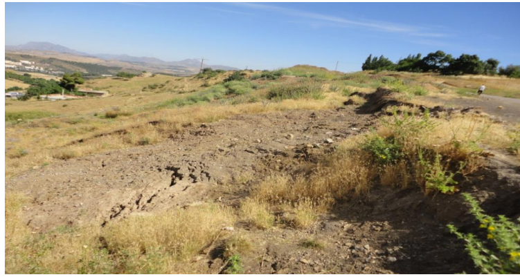
Photo.VI.6 : Glissement de Ouled Fayed.
