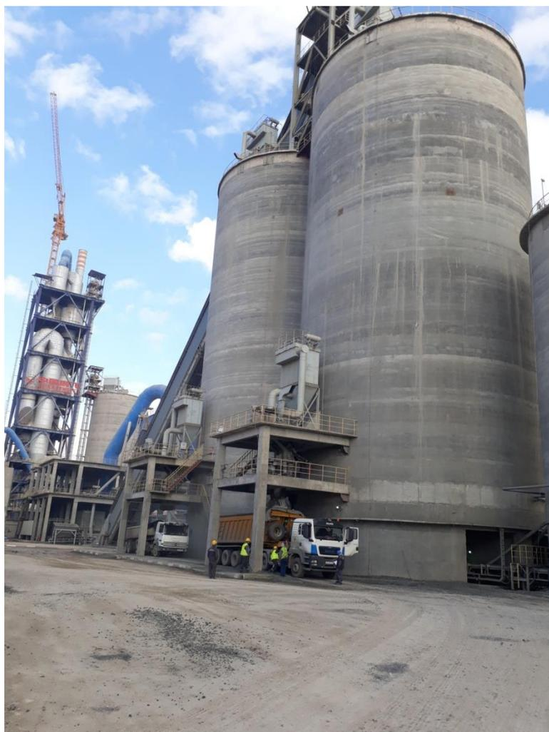
**Figure I.15 Silo stockage de clinker[1]**
