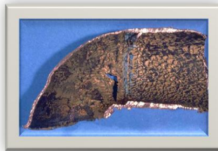
Figure 28 - La corrosion caverneuse.
