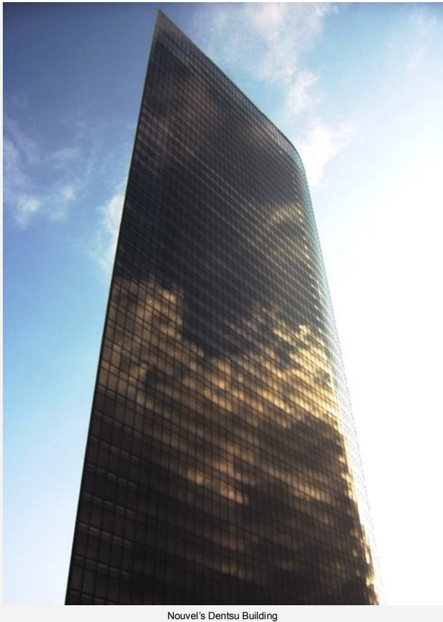
Nouvel's Dentsu Building
