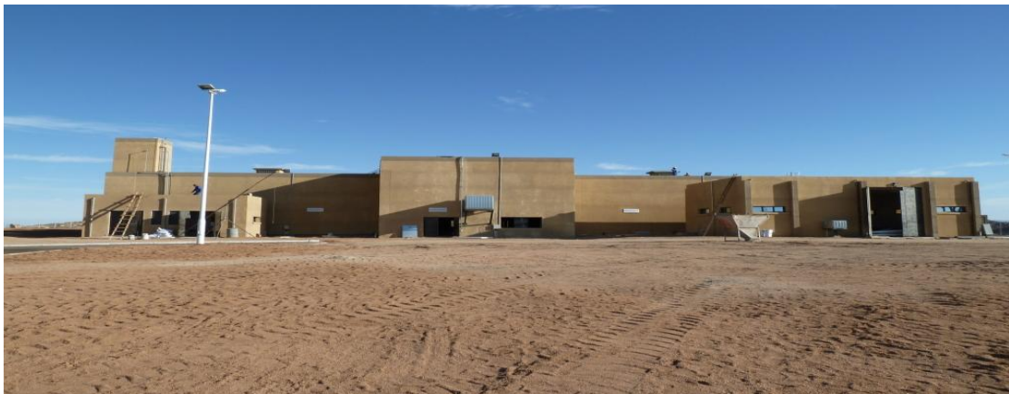
Figure (I.7) Station de pompage n 06
