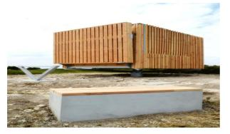
**Figure 1.14:** The Figuerolles Park had a temporary lookout, exposed to the wind and solar radiation, disassembled at the end of the season, each year. Intended to accommodate two guards during the summer season.
