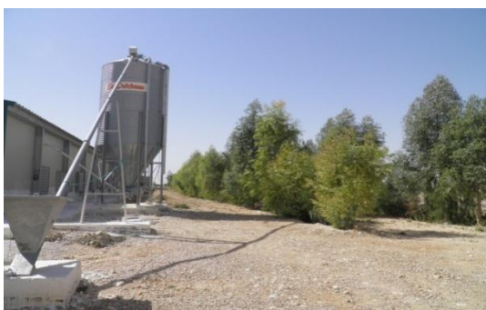
Figure 16: Le silo(photo originale,2019)
