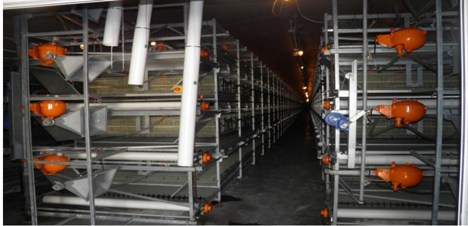
Figure 15: Les batteries(photo originale,2019)
