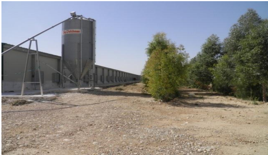
Figure 13 : Brises vents(photo originale,2019).
