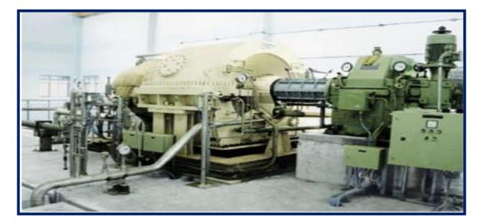
Figure 45: Roi ET, Thailand: Turboset for the Bua Sommai Electricity biomass power plant.
