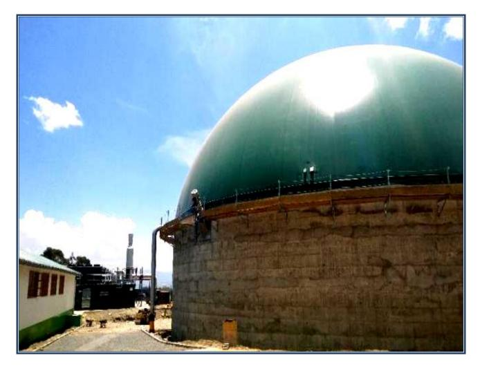
Figure 07: A biogas digester.
