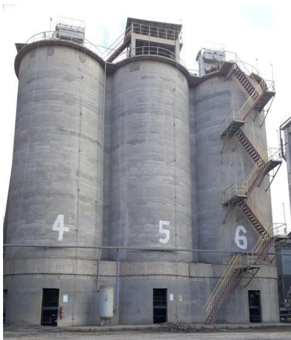
Figure I.18 : Silo stockage de ciment.
