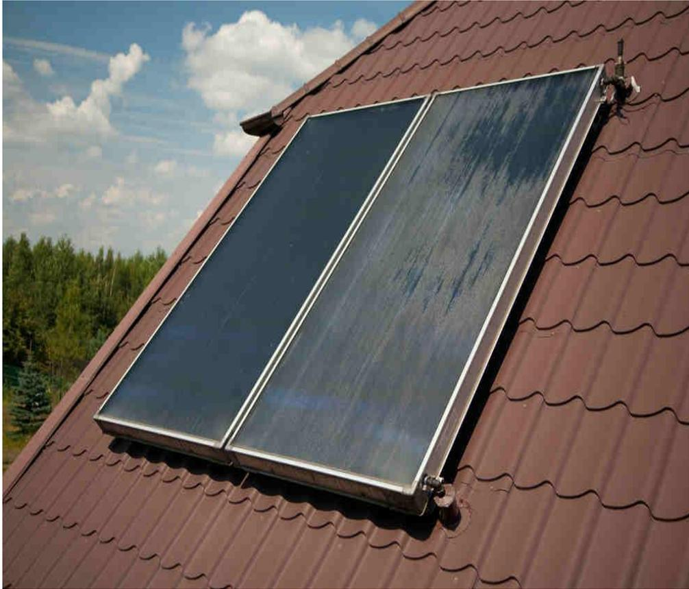
**Figure I.1 :** Flat plate solar collector.
