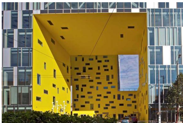
Figure 61. Saint-Etienne office building
