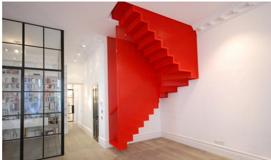
Figure 59 Bespoke red hot perforated steel suspended staircase
