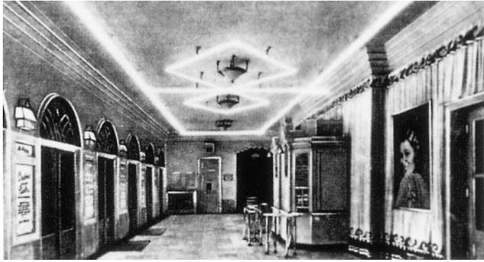
Figure 33. Theatre foyer lit by Moore lamps.
