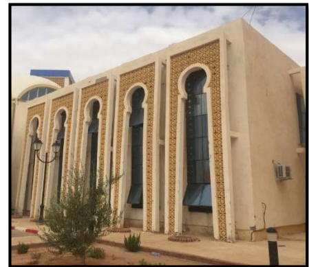
Figure 118 The External Arcs Structure - source: Student Photography
