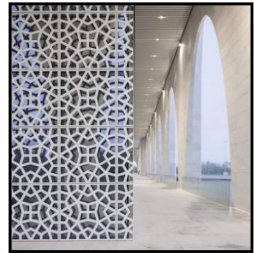
Figure 61the External Envelope- source : www.archdaily.com
