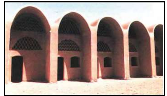
Figure 77 the Using of Arcades to protect the openings in Egypt - source: (Bader Eddin Elkhoul, 1975)
