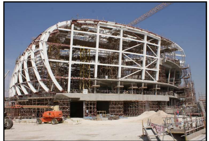
Figure 38 QFIS Structural system Roof Steelwork- source: www.constructionweekonline.com
