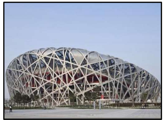
Figure 63 the envelope of Bird's Nest Stadium - China- source: www.Archdaily.com
