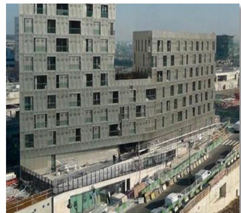
Figure 85 : rue et entrée l'ilot M9D4 Source: architizer.com/projects/m9d4-
