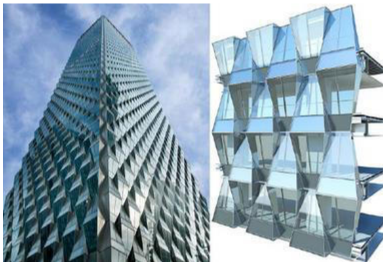
Figure 32: centre de green land – Pékin / module d'auto-ombrage inspiré de l'origami (Source : https://www.slideshare.net/roopachikkalgi/shading-devices- )
