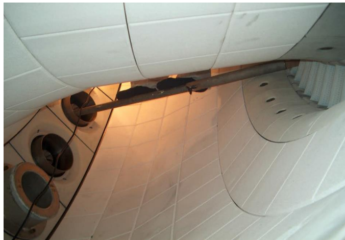
Figure I-13: La chambre de combustion.
