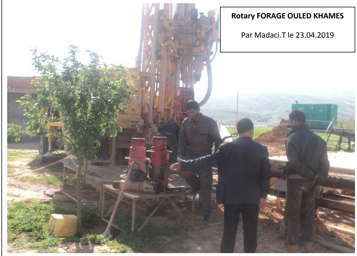
Figure 09 : Forage rotary circulation direct
