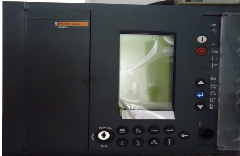
Figure III.11 : Relais de protection sepam.
