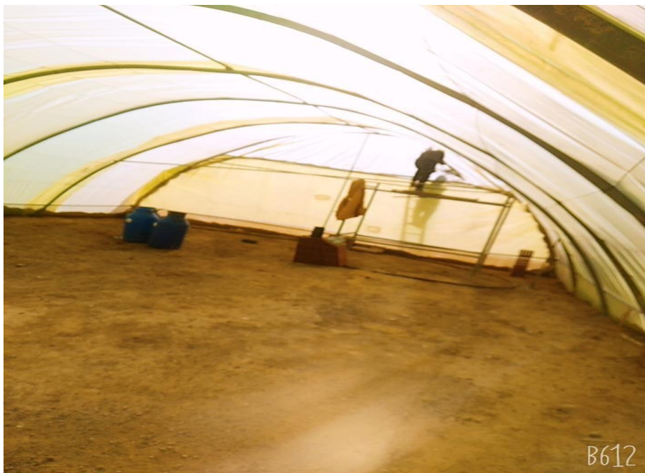
Figure 05 : Installation de la serre (Original)
