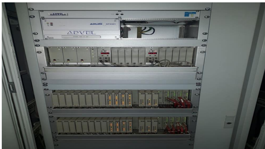
Figure I.24. Armoire ESD.
