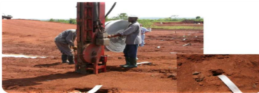
Figure I.10 Installation des drains verticaux [20].
