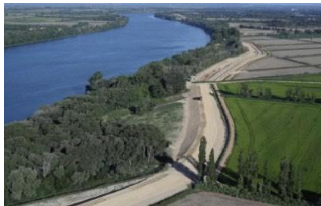
Figure II.6: Ouvrages de protection des inondations
