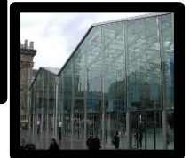
Figure 24La façade VEA
