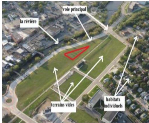
Figure 83: la situation de muséewisconsin source :google earth
