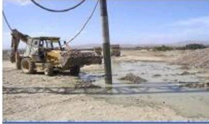
Figure II.22: introduction du ballast (22)
