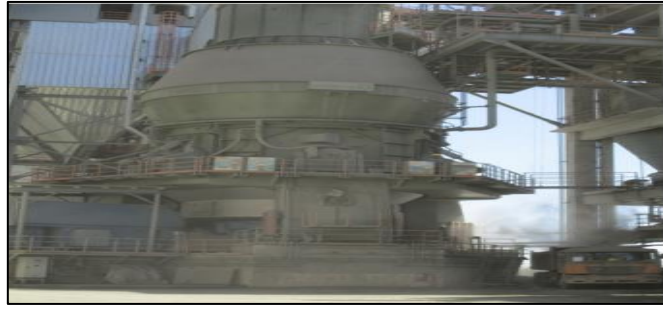
Figure I.22: broyeur de ciment VCM
