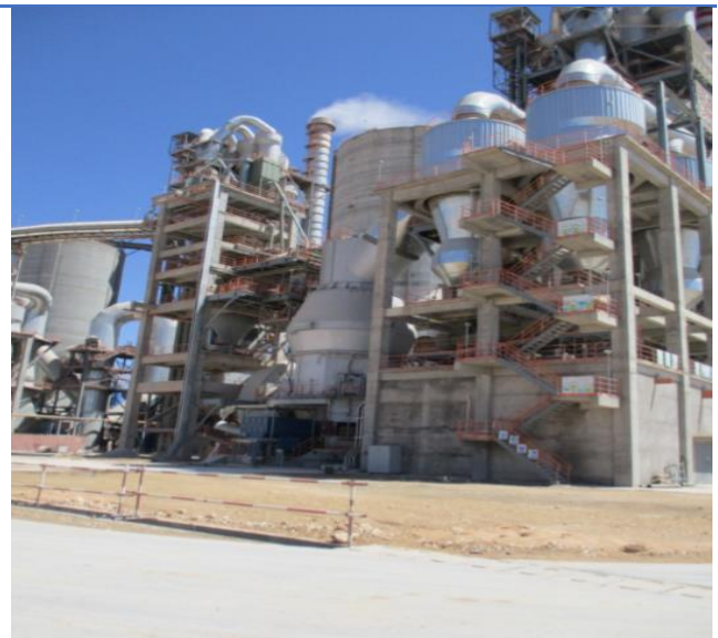
Figure I.17 Broyeur cru.
