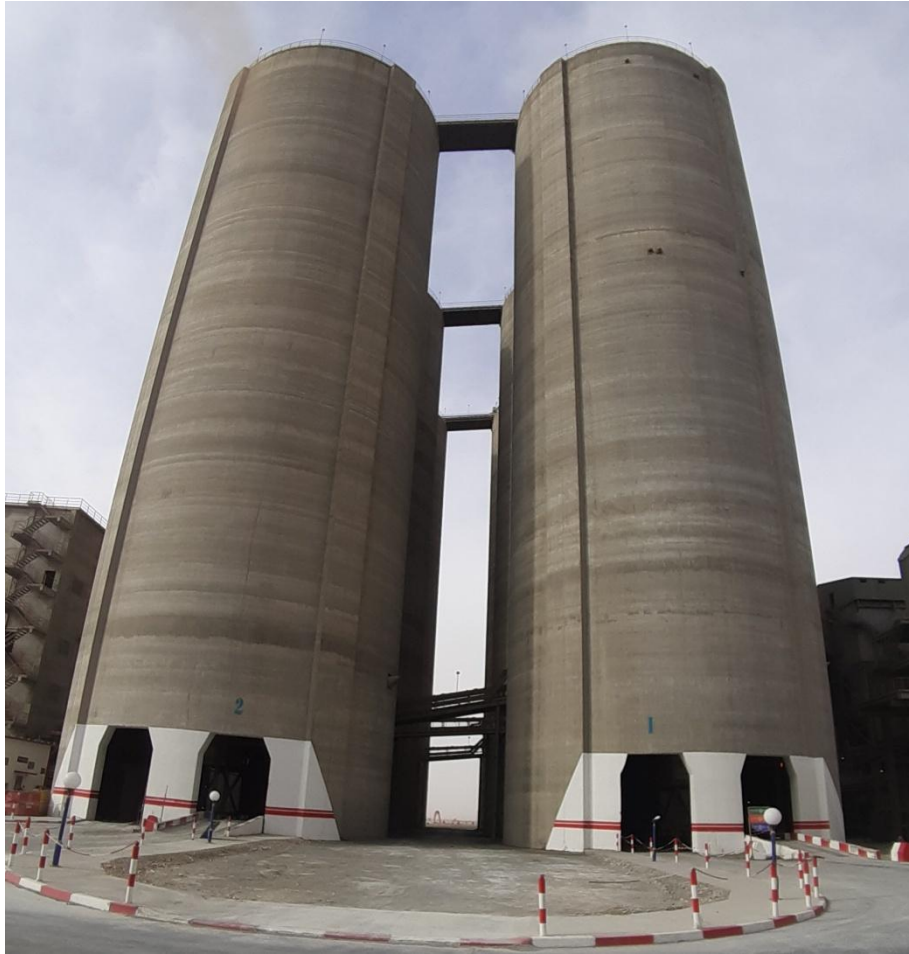
Figure I.14: Silo stockage de ciment.
