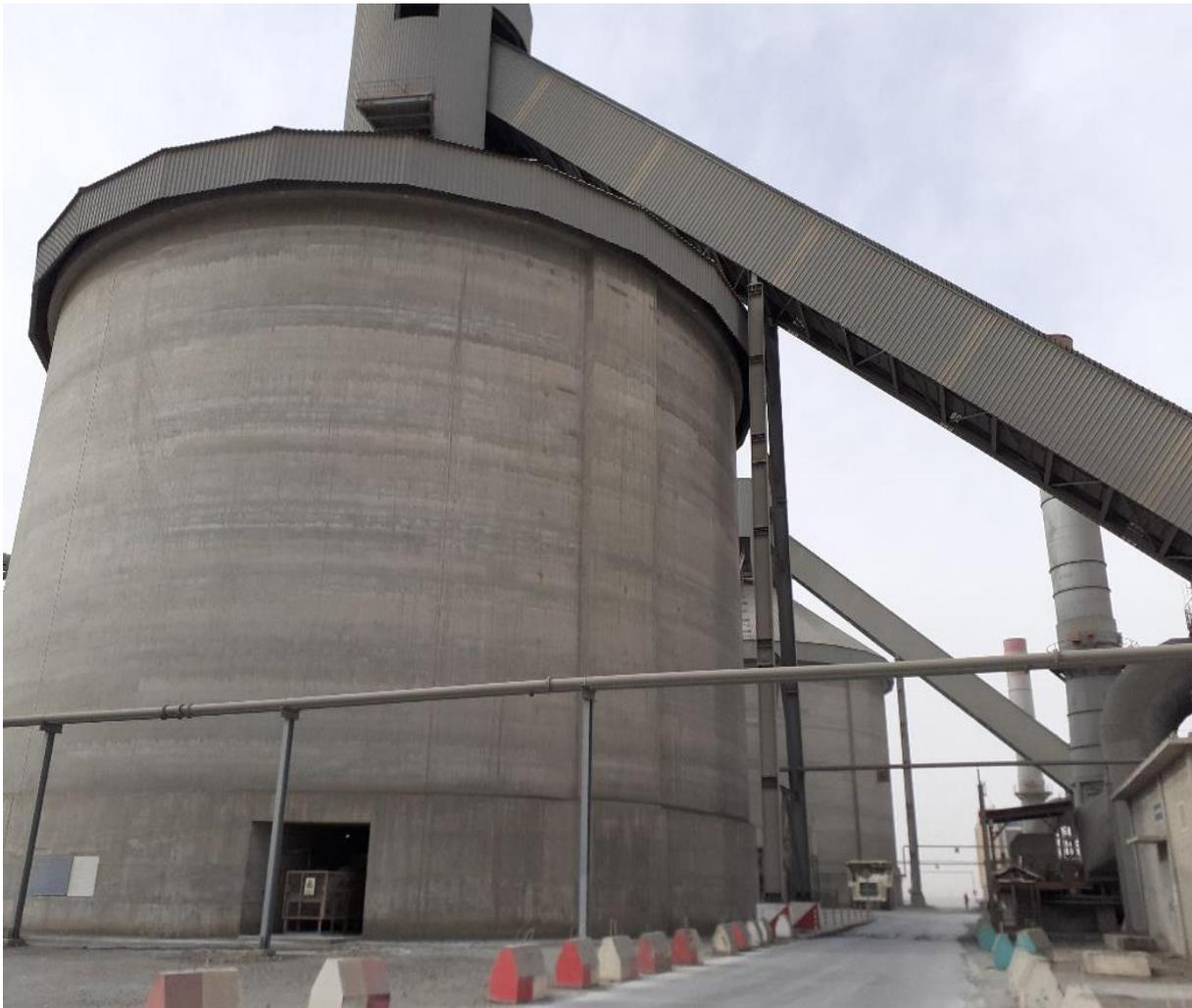
**Figure I.16:** Silos stockage de clinker.
