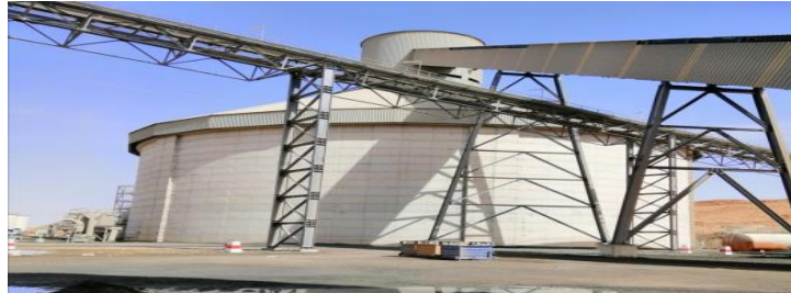
Figure II. 8 : Silos stockage de clinker. [11]
