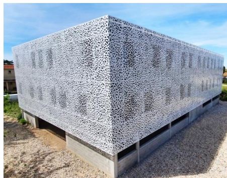
Figure 23: enveloppe multicouche Source : france-resille.com
