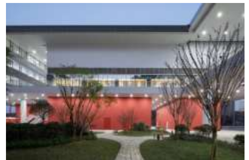
Figure 78: Courtyard Source: www.archdaily.com
