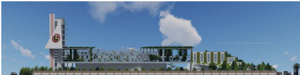
Figure 177: Southern façade Source: author
