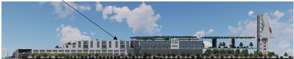
Figure 180: Western façade Source: author
