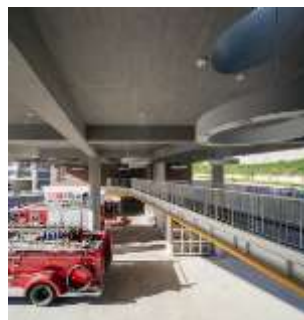
Figure 92: Parking Area And bridge Source: www.archdaily.com
