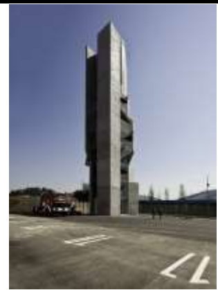
Figure 12: Textured Tower, 2012, training tower. Source: www.archdaily.com
