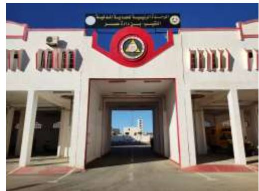
Figure 97: front view, main unit civil defense biskra Source: Author 2022
