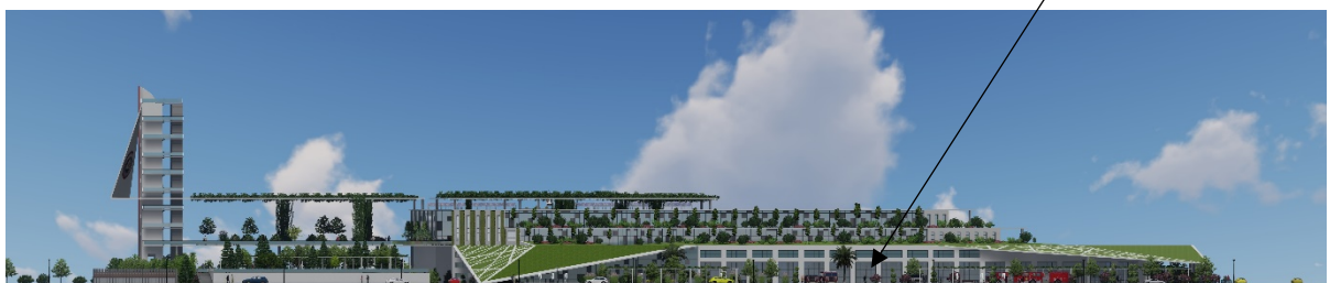
Figure 178: Eastern façade. Source: author
