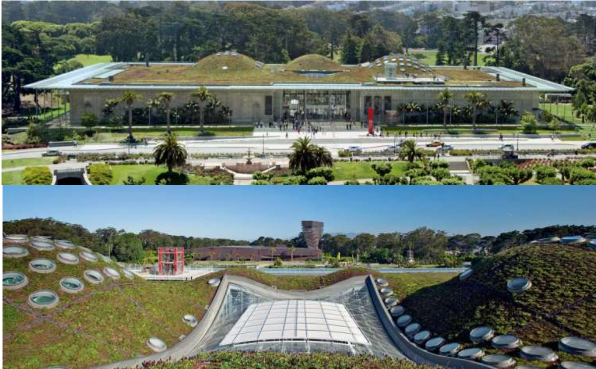
Figure 25: Renzo Piano Building Workshop, California Academy of Sciences, San Francisco, USA, 2008, exterior and roof Source: Sayigh, A., & Trombadore, A. (2021).
