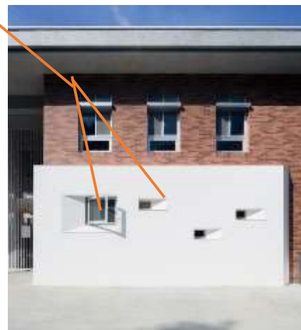
Figure 86: front facade , right Source: www.archdaily.com
