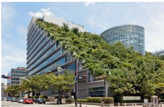
Figure 28: Emilio Ambasz and Associates, ACROS Building, Fukuoka, Japan, 2000. Source: Schröpfer, T. (2022).
