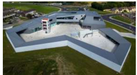
Figure 44: Aerial View, Waterford station Source: www.archdaily.com
