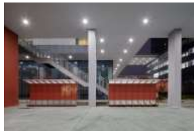
Figure 76: Fire Truck Parking Space Source: www.archdaily.com
