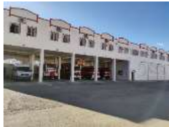
Figure 111: Apparatus bay/Equipment Storage
