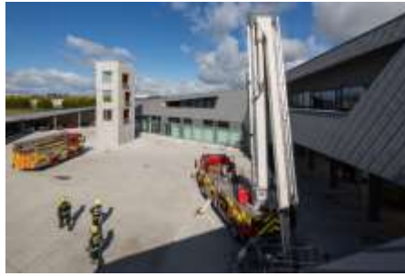
Figure 56: Training Yard Source: www.archdaily.com
