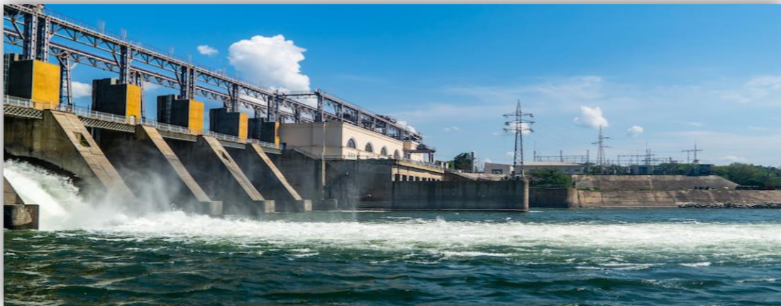
Figure I.13: La centrale hydraulique
