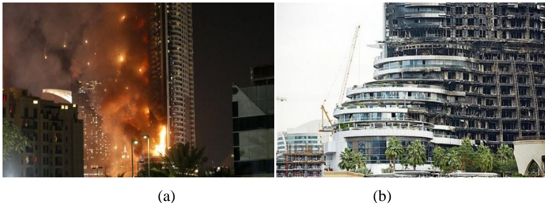
Figure I.7. (a) Address downtown hotel during the fire, (b) Address downtown hotel after the fire.
