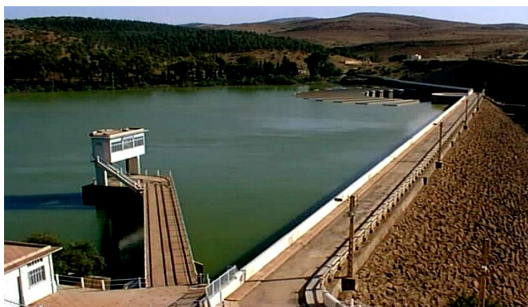
Fig. III.16 : Barrage de Ghrib, Ain Defla ( http://www.algermiliana.com/medias/images/84729769-o )
