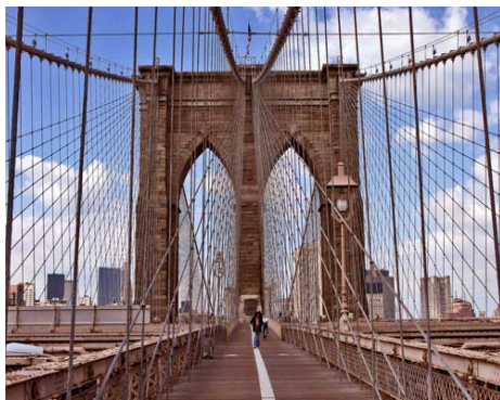
Fig.1.1 Brooklyn bridge New York 1883
