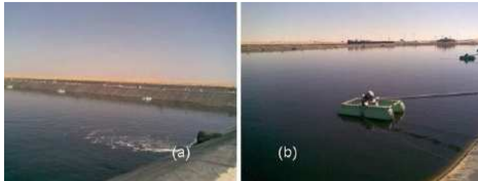
Figure 2.20 – Lagunes en service.
