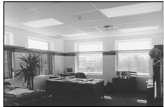
Figure 38 : Le système light shelf. (Source: ENERGY EFFICIENCY MANUAL, CONTROL AND USE OF SUNLIGHT)
