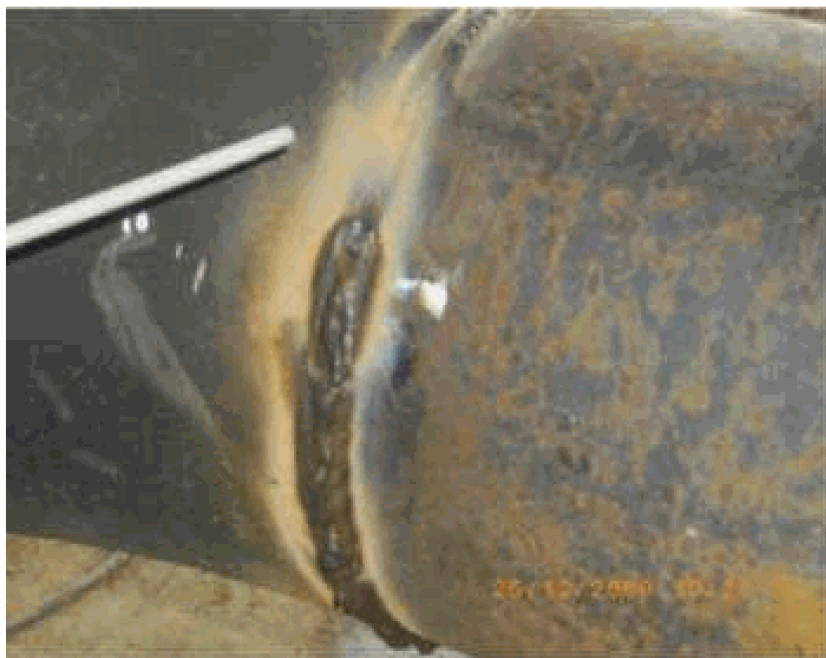
Figure.III.1: X70 pipeline steel after industrial arc welding.
