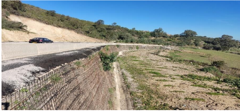
Figure 1-7 Mur en sol renforcé wilaya de Jijel.
