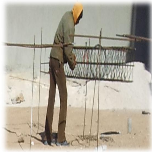
- Ferrailage poteaux-
